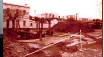
This high pressure 153 km pipeline ran from Altona to Western port was commissioned in 1972. The 24 inch pipeline ran along Richardson Street. The construction works were massive, causing access problems and disruption to local residents. Problems were encountered when excavation works went below the water table.
